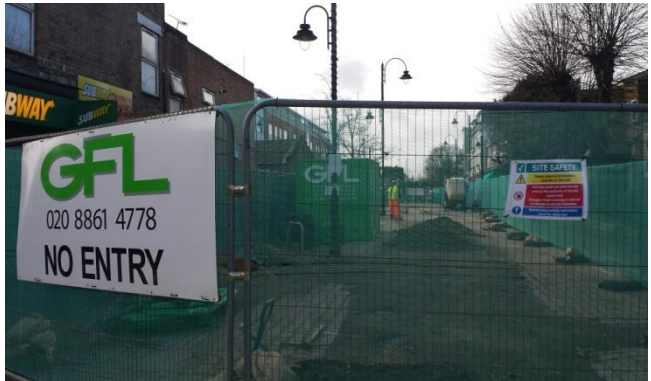
Works at Wealdstone Square
